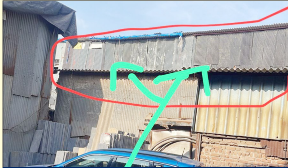
Ward No 168, Contractor Ragga , Owner Ram Seth Tyre Waala...Site Add: Munna Seth Compound, Nr Manohar Garage, Before Maharashtra Kaata, Sion-Kurla Link Road, Kurla W
